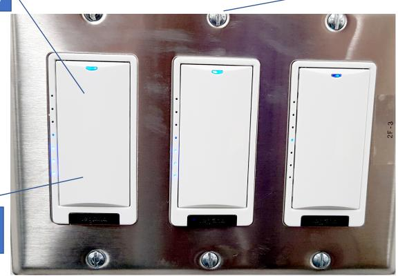
Press the bottom part of the switch to turn off and decrease the light intensity
